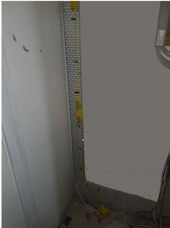
Figure 4: Examples of Vertical Telecommunications Pathways
